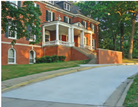
New concrete driveway installed
